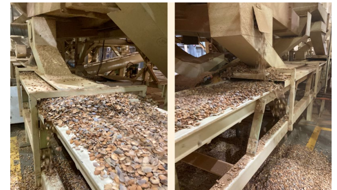
Kernel Conveyance capacity upgrade
